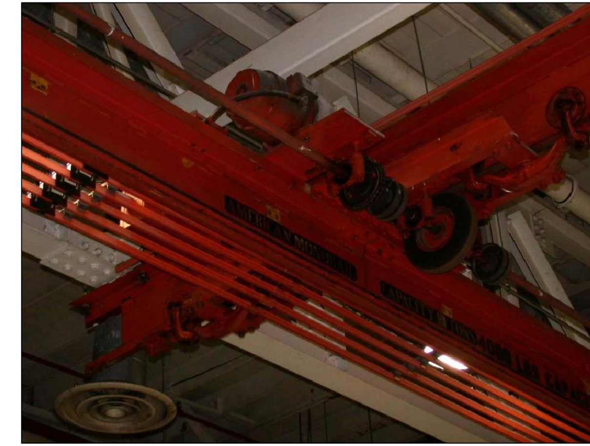
B PICTURE - EXISTING BRIDGE DRIVE (WHS #165 AND WHS #205) 4 5 SCALE: NTS
