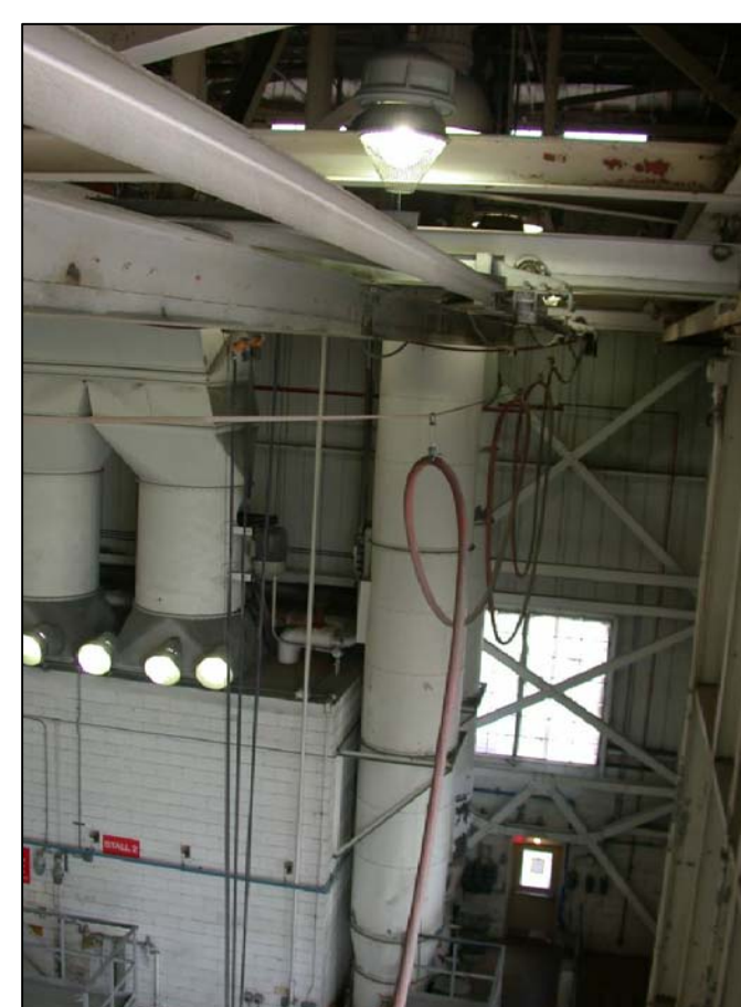
E PICTURE - EXISTING AIR HOSE AND FESTOON SYSTEM NOT TO SCALE
