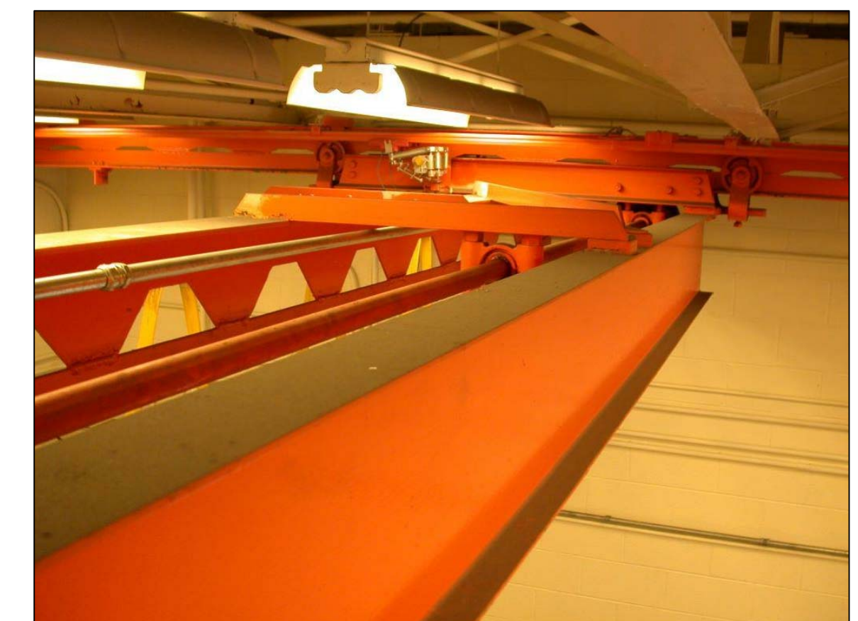
C PICTURE - EXISTING BRIDGE CRANE SCALE: NTS
