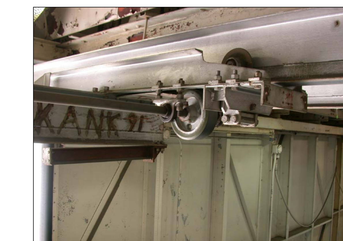
C PICTURE - EXISTING BRIDGE TRUCK NOT TO SCALE
