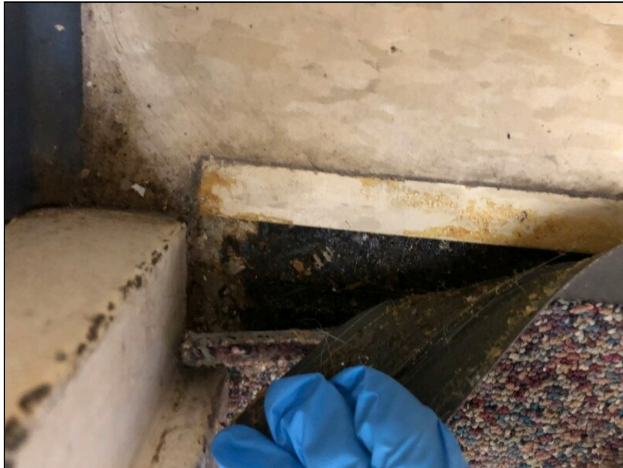
3 - View of Black Mastic Under Carpet
