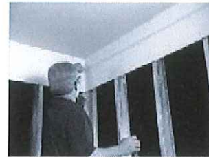
Mark desired height for new ceiling
