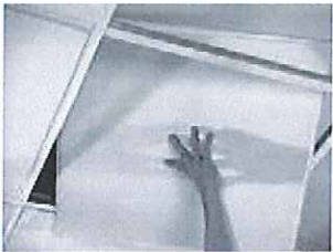
Tilt panels above frame and drop into place
