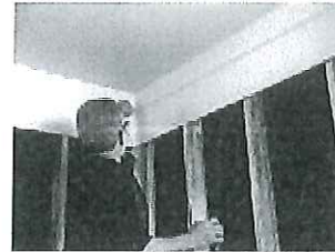
Mark desired height for new ceiling
