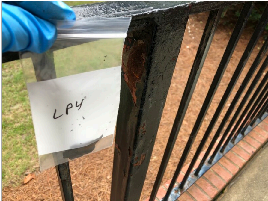
13 - View of Lead Paint (Sample LBP04), lead paint not detected
