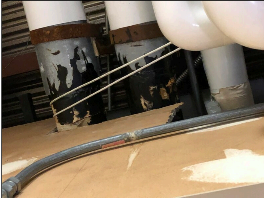
5 - View of TSI, Ceiling Tiles, and Black Caulk
