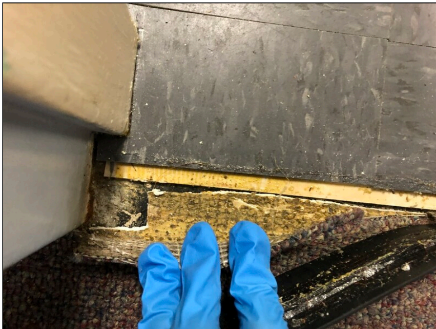
2 - View of Carpeting, Black Mastic, Black Tile, and Yellow Mastic
