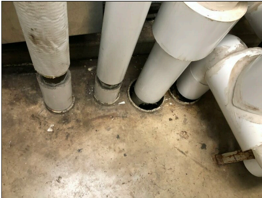
4 - View of TSI and Pipe Elbows
